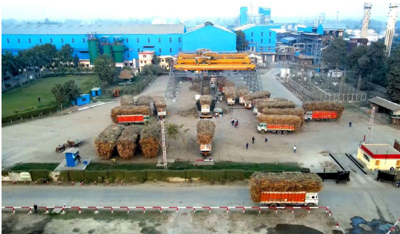
Aerial view of sugar plant, DN unit
