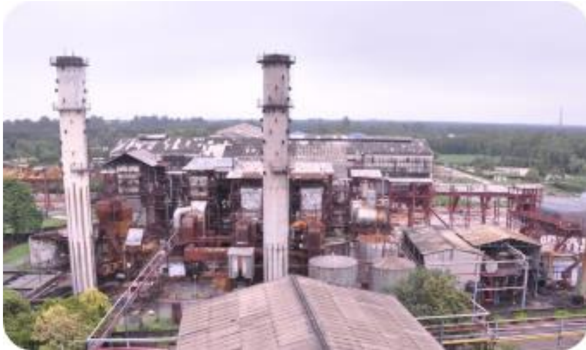
Sugar Plant Overview
