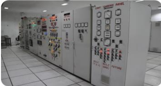
Cogeneration Control Panel
