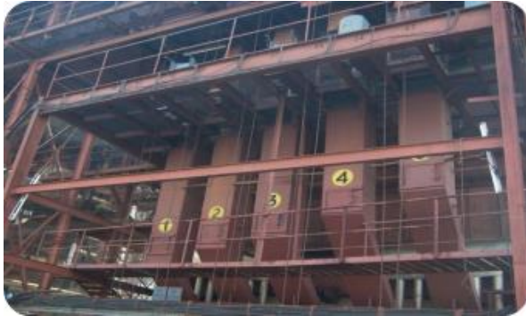
Bagasse Silos & Feeders of Boiler
